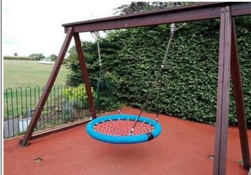
**Finding:** The orientation of the swing joints are not in the direction of travel and this can lead to excessive wear
