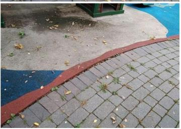
**Finding:** The surface is lifting at the edges and creating trip **Action:** Repair perimeter of surfacing to remove trip points points
