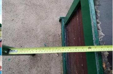
**Finding:** The fireman's pole is less than 350mm from the platform and fails to meet the recommendations of BS EN 1176 Part 1
