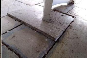
**Finding:** The slab is lifting at the edges and creating trip points
