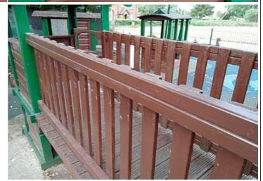
**Finding:** The design of the barriers encourages standing or **Action:** Monitor - No remedial work recommended sitting and fails the requirements of BS EN 1176
