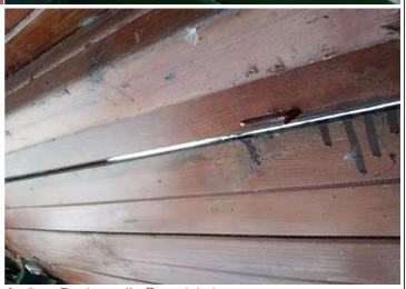
**Finding:** There are areas or parts of the timber roof on the structure that have rotted **Action:** Replace all affected timbers
