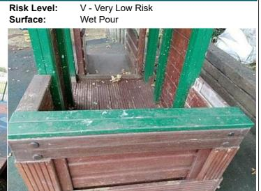
**Finding:** The design of the barriers encourages standing or **Action:** Monitor - No remedial work recommended sitting and fails the requirements of BS EN 1176
