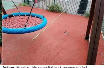
Finding: BS EN 1176 requires an additional 0.5m of unobstructed space at each end of the swing surfacing area. This is a relatively low risk finding and no remedial action is recommended at this point.
