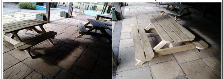
**Finding:** The bench is not securely fixed to the surface and **Action:** Secure the bench to the ground there is some possibility of the item tipping or rolling over
