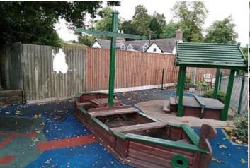
**Finding:** The shelter forms a hard object within the impact area of the equipment in contravention of the requirements of BS EN 1176 Part 1
