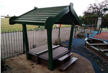
Finding: There are areas or parts of the timber roof on the Action: Replace all affected timbers structure that have rotted
