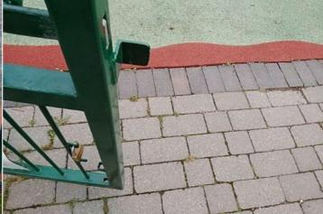
Finding: The rubber buffer is missing from the latch plate
