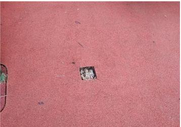
**Finding:** The surfacing is severely damaged exposing the concrete underneath
