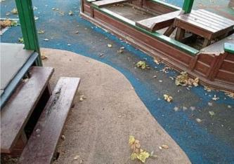
**Finding:** The boat forms a hard object within the impact area of the equipment in contravention of the requirements of BS EN 1176 Part 1
